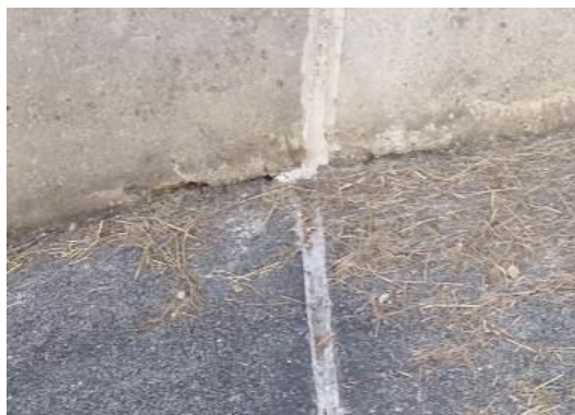
Erosion bajoyer 3 e joint aval passerelle RD
