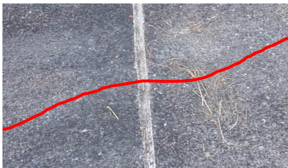
Erosion bajoyer 3 e joint aval passerelle RD
